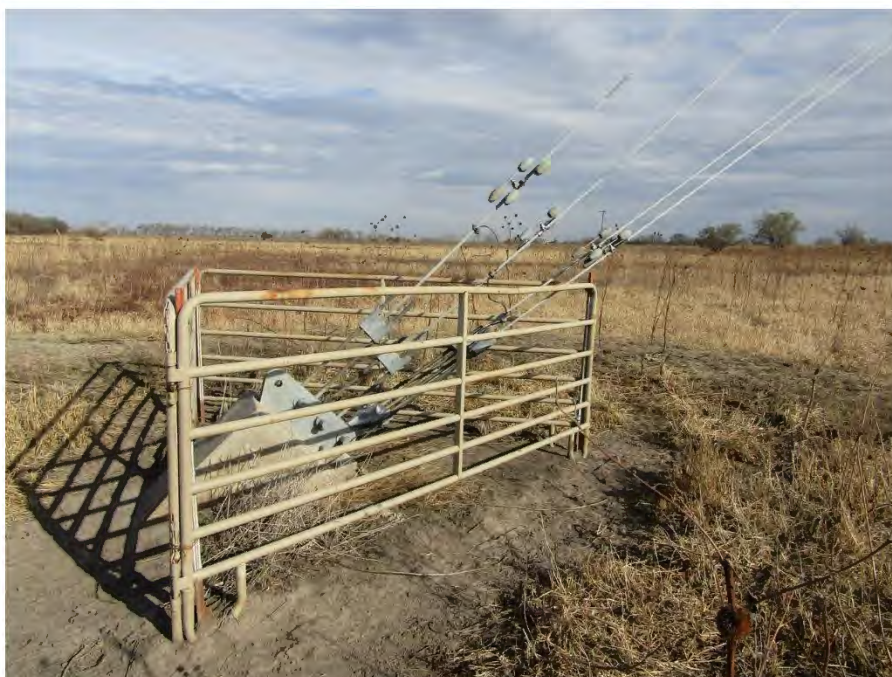
Typical fencing at the anchors, and dampers on the guy wires.
