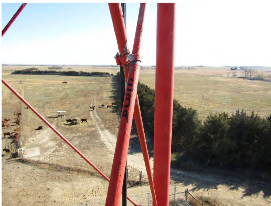
Typical loose banding at the intersection of diagonals.
