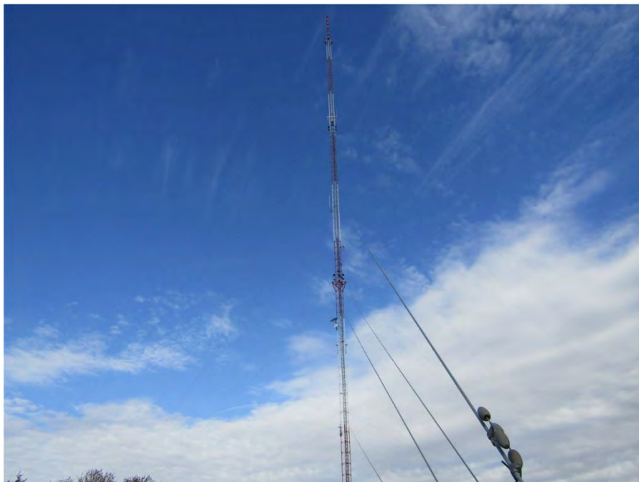
Profile view of tower.
