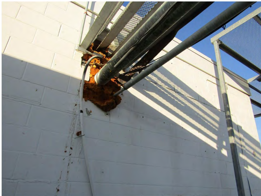
Transmission line entering the building.
