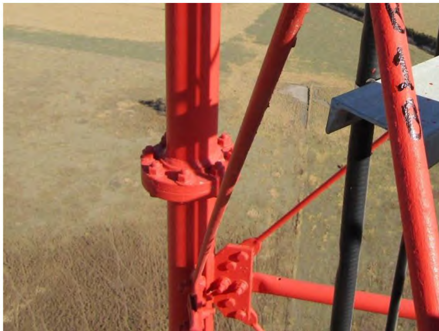
Typical leg splice and gusset plate connections.
