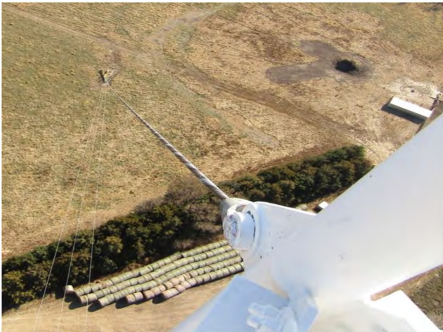
Typical areas of surface rust on at the upper end of a level #3 guy wire.
