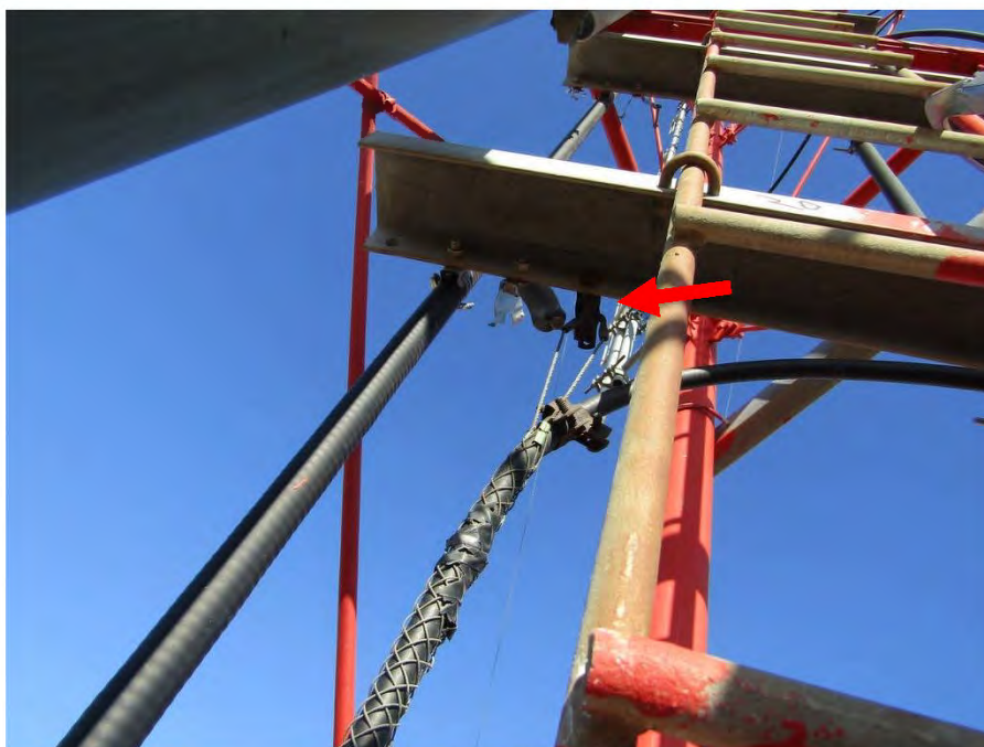
Hoisting grip for the flexible line feeding the dipole antenna in section #20 secured with a butterfly clamp.
