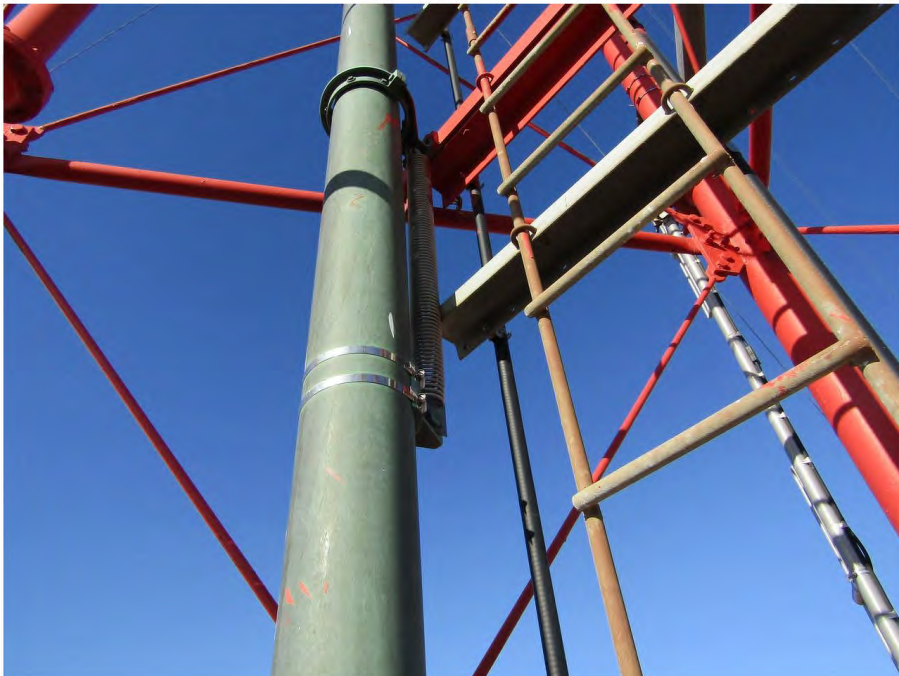
Typical spring hanger. Photo also shows surface rust on the ladder.
