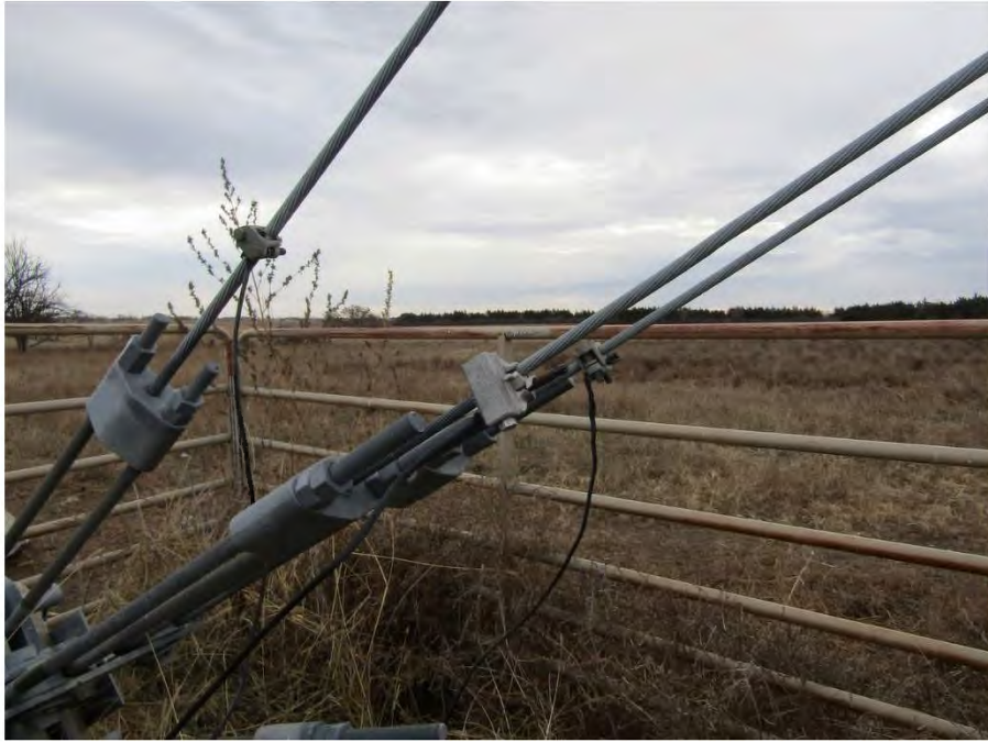
Typical grounding cable connections on guy wires.
