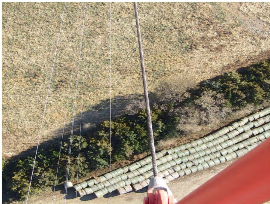
Typical areas of surface rust on a level #5 guy wire.
