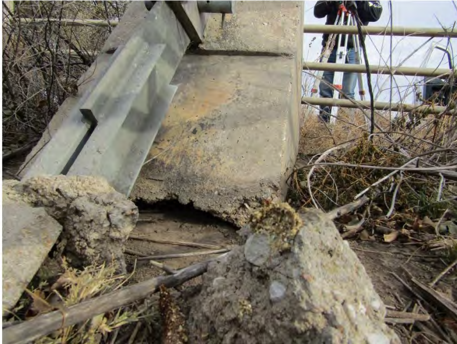
Broken concrete at the outer anchor A.
