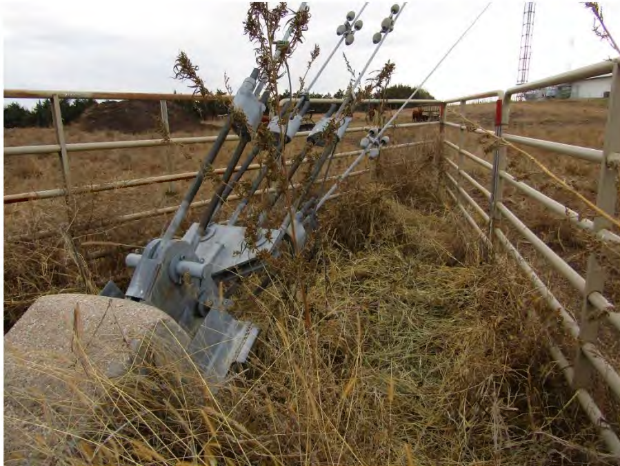
Inner anchor A with brush growing on the guy wires.
