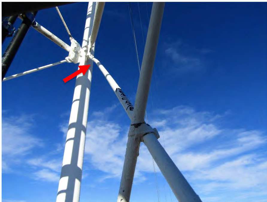
Bend at the upper end of diagonal member in Section #15.
