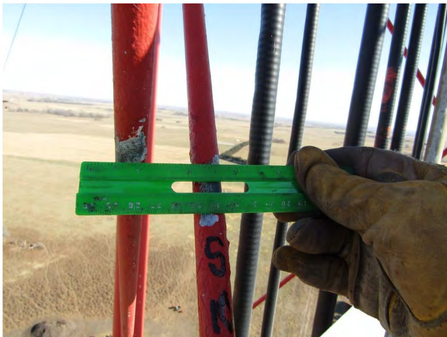
Typical missing banding at the intersection of diagonals.
