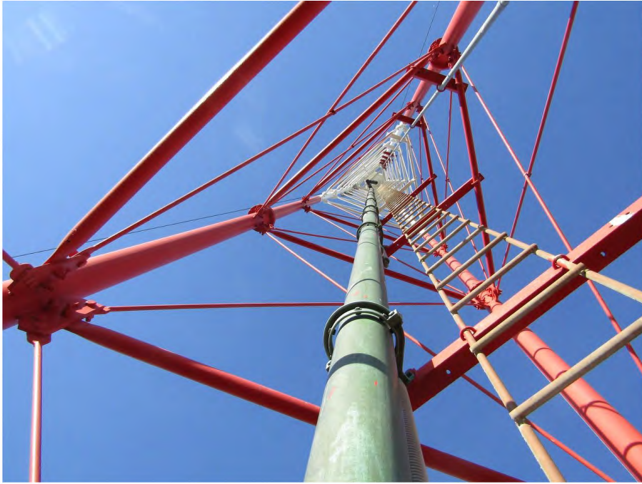
Transmission line location in the tower.
