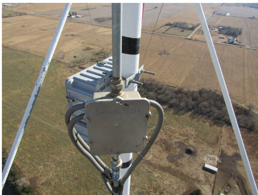
Junction box at light level #2.
