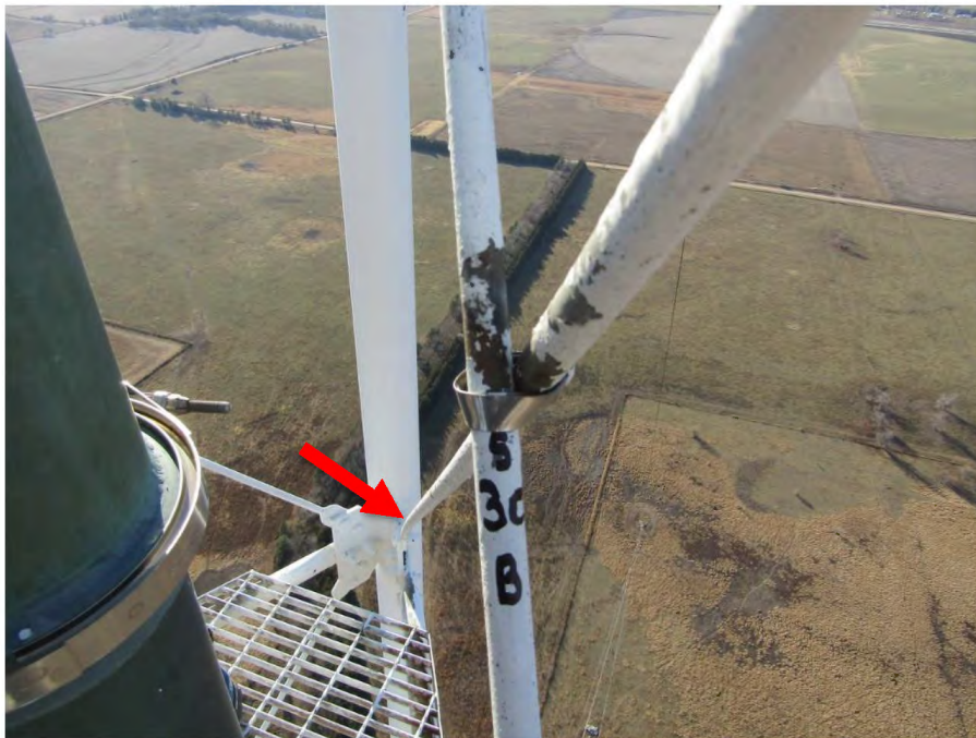
Bent diagonal member in Section #30. Photo also shows loose banding and surface rust at the intersection of the diagonal members.
