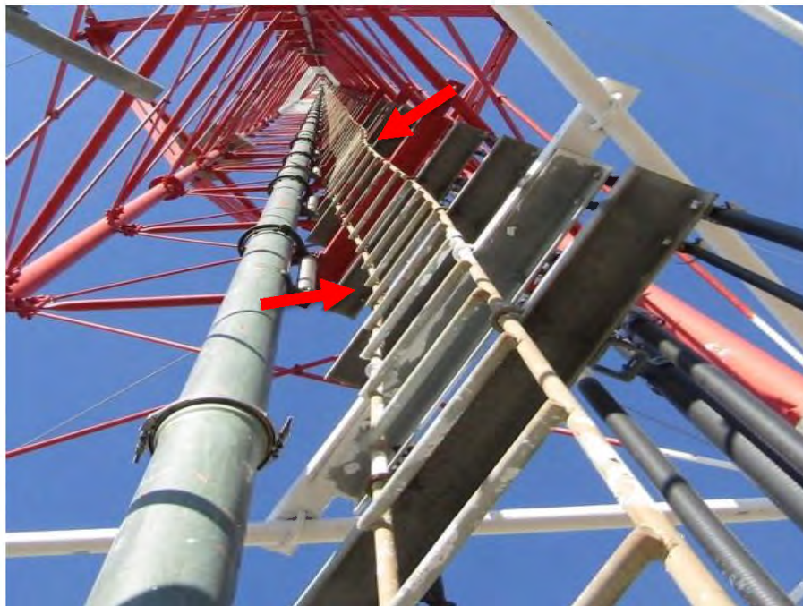
C-channel mounting brackets secured to the ladder below guy level #2. Photo also shows two significant bows in the ladder.
