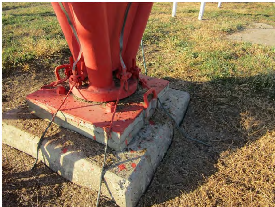
Grounding at the tower base.
