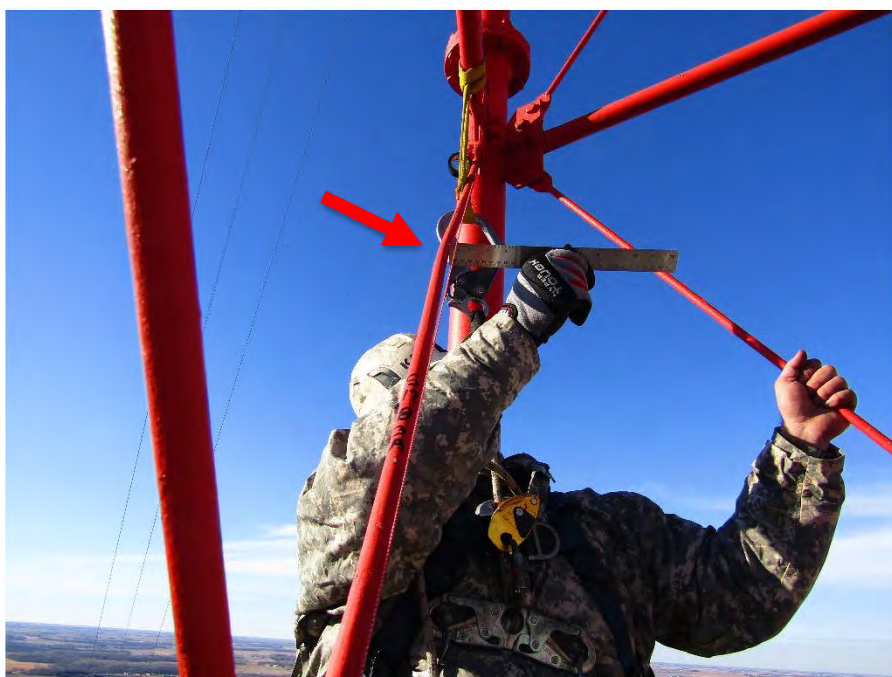
Bent diagonal member in Section #17.
