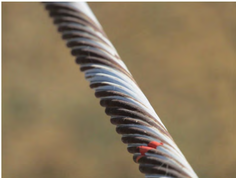
Typical areas of surface rust on a level #3 guy wire.
