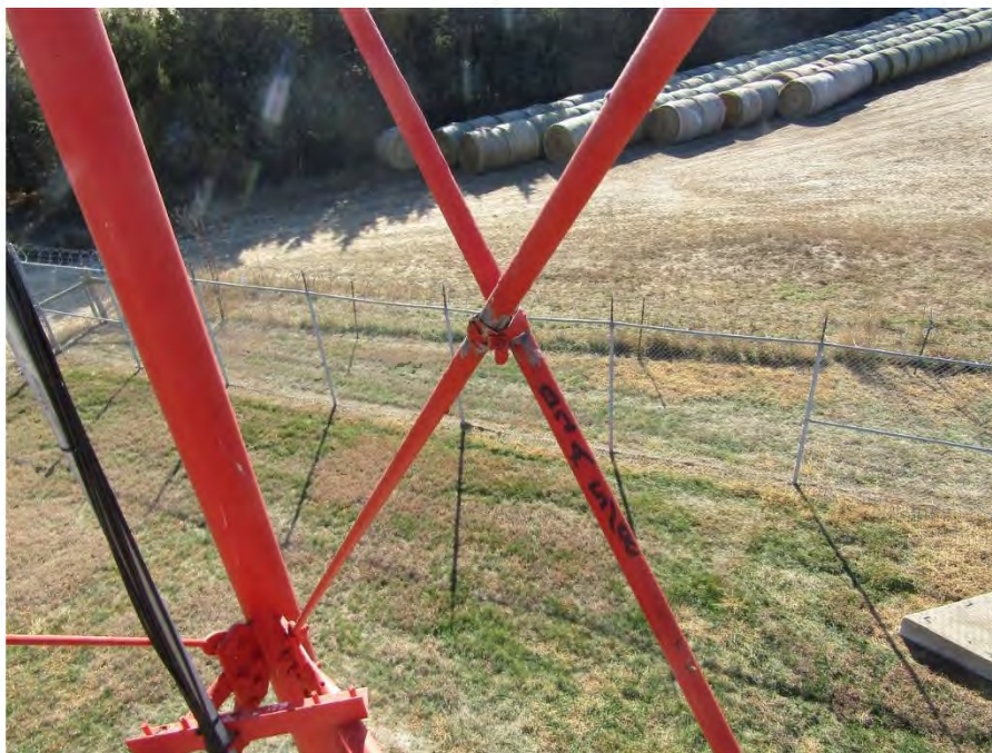
Typical loose banding at the intersection of diagonals.
